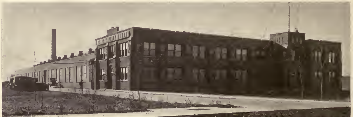
VIEW FROM NORTHEAST BUILDING FOR WALKER VEHICLE CO., CHICAGO, ILL. GEORGE C. NIMMONS & CO., ARCHITECTS
